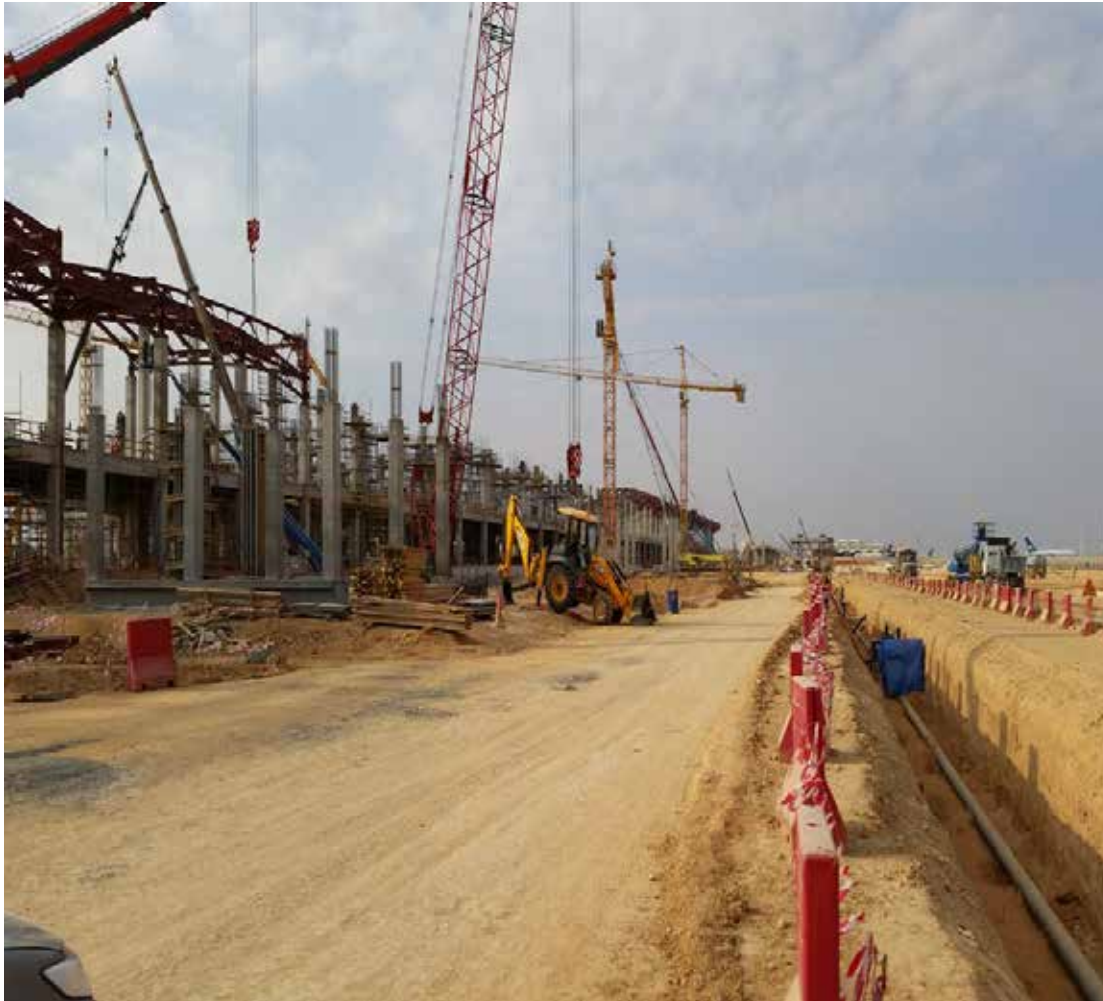
A view from Construction Site of Riyadh Airport, KSA Terminal-5 Building
